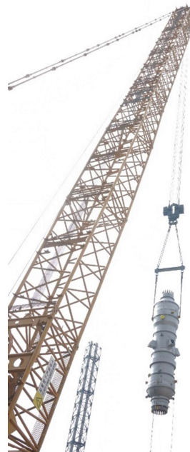
HP Stripper unloaded from vessel and transported by road to PPL, Mangalore
