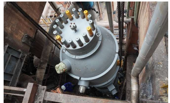
HP Stripper erection
