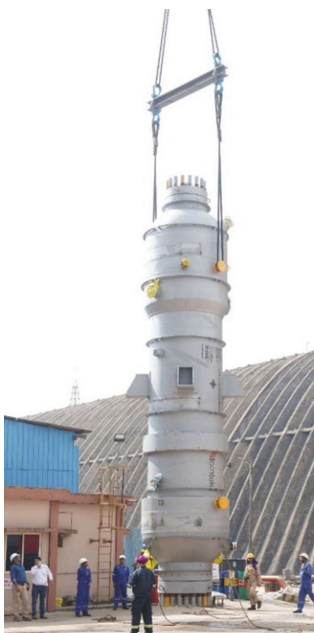
HP Stripper unloaded from vessel and transported by road to PPL, Mangalore
